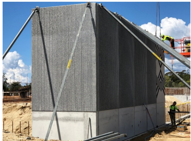
Photo above - Starting the exterior wall
